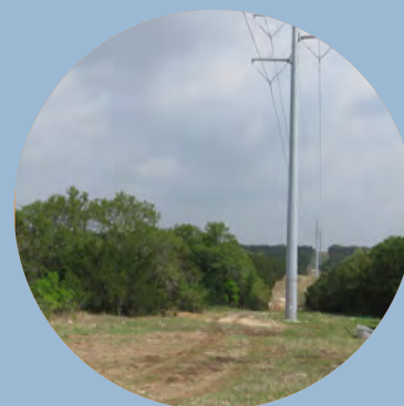
Utility Service Access San Marcos, TX
