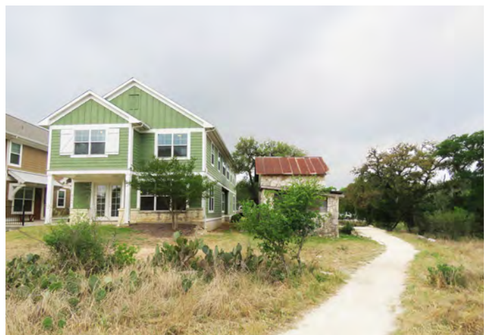
IMPROVING WILDFIRE MANAGEMENT STRATEGIES IN THE WILDLAND URBAN INTERFACE WILL REDUCE RISK TO ABUTTING DEVELOPMENTS
